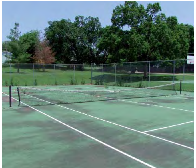
Image 2: The tennis court is unusable due to the decayed net, uneven surface, and weed growth
