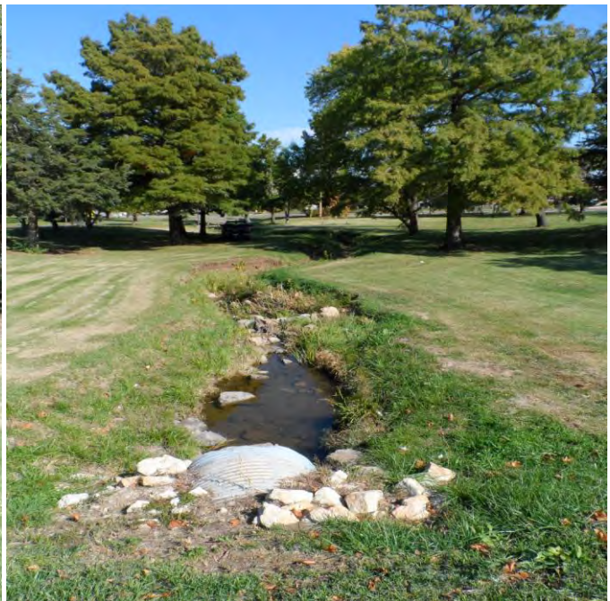
Image 4: Drainage ditch has cut away the stream bank and needs to be remediated to slow down runoff and improve erosion of the ditch.
