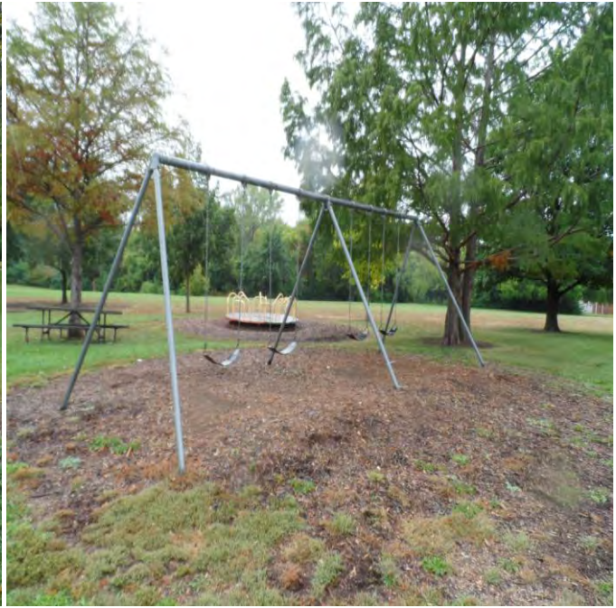
Image 2: Existing swing set that does not have an accessible route or surface.
