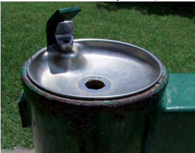
Image 3: Water fountains on the site are corroded and hazardous to human health
