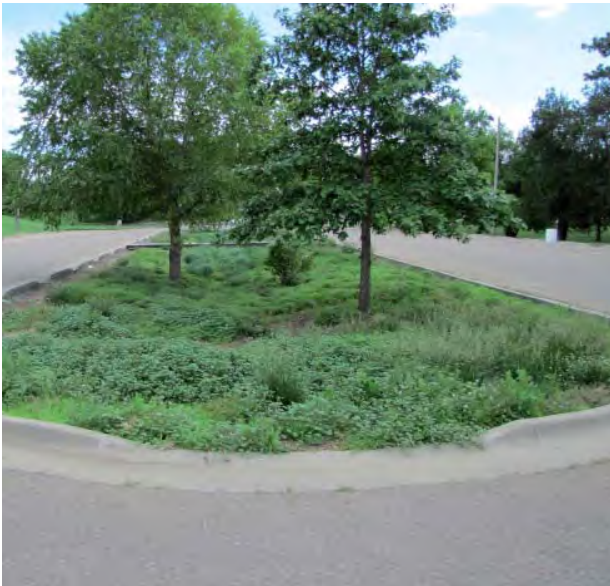
Image 1: Bioswales provide good management of rainwater and enhance the site's visual character
