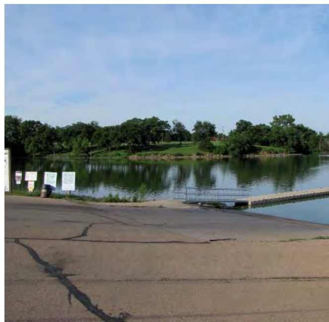
Image 4: Paving around the south boat ramp and marina needs to be re-surfaced
