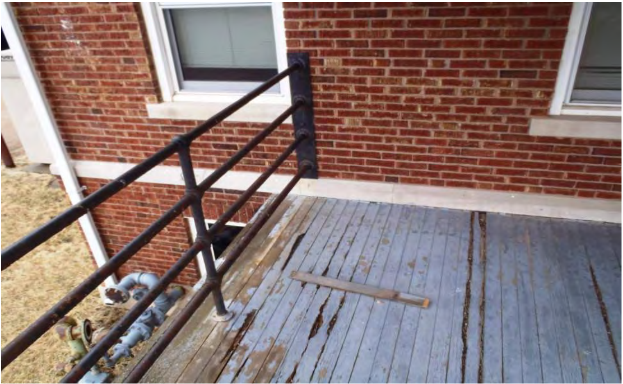
Photo FG - West Deck Deterioration
