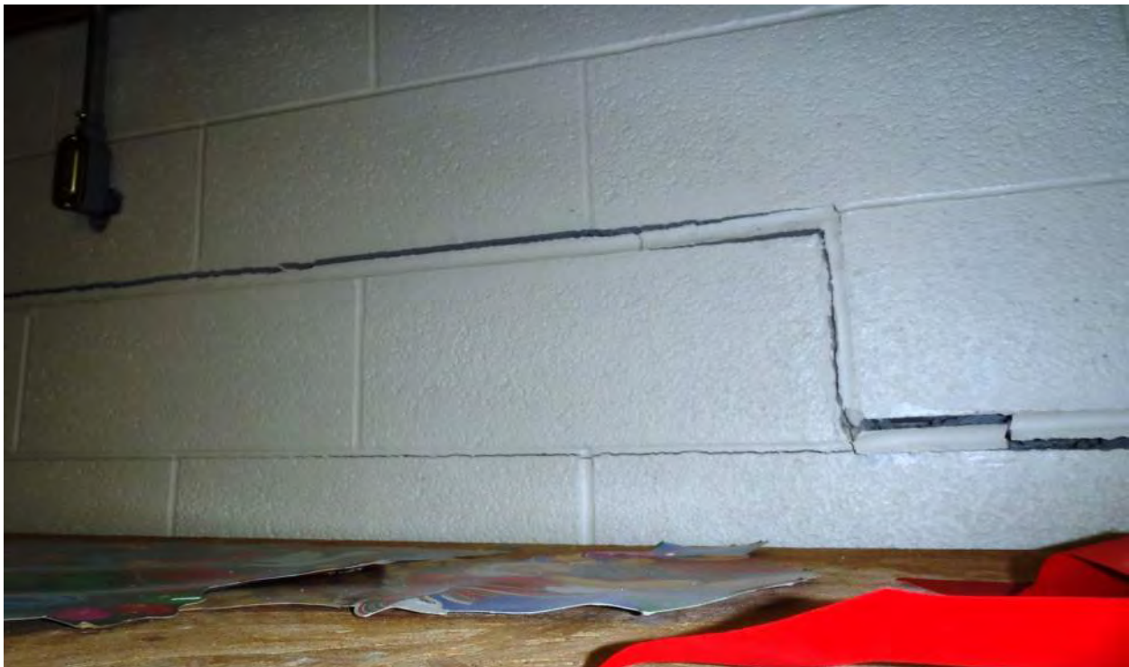
Photo 7A - Significant Wall Crack at Mechanical Room Masonry
