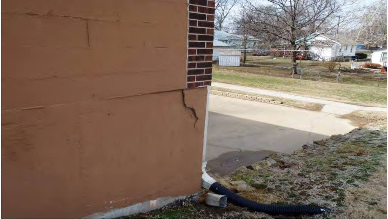
Photo 7E - Concrete Crack / Spall at Lower Level
