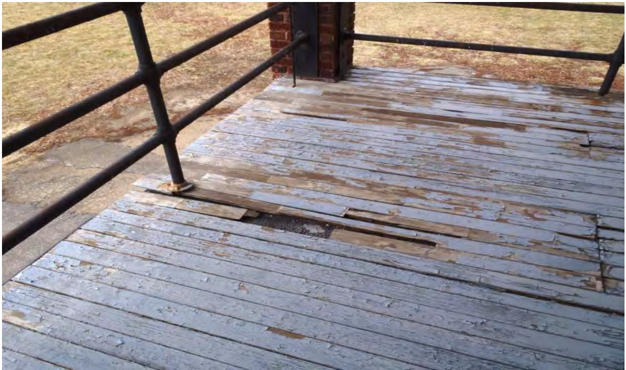
Photo 4C - West Deck Deterioration
