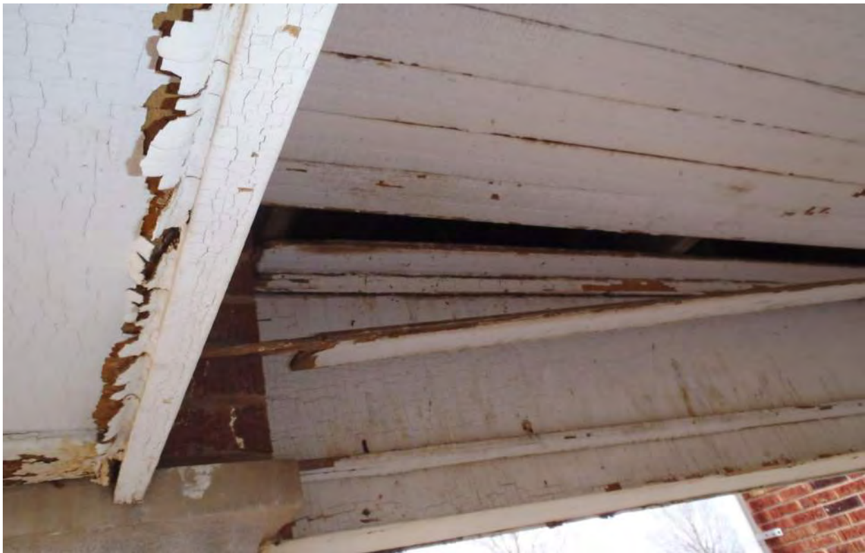
Photo 4F - West Deck Deterioration
