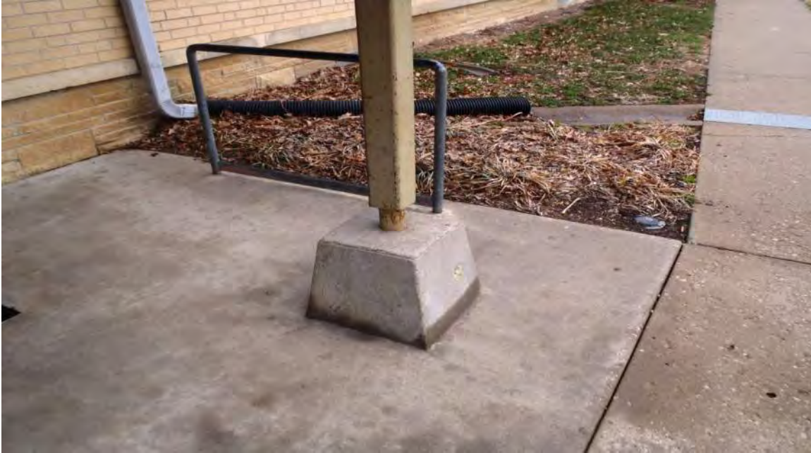
Photo 2A - Minor Corrosion at Exterior Column
