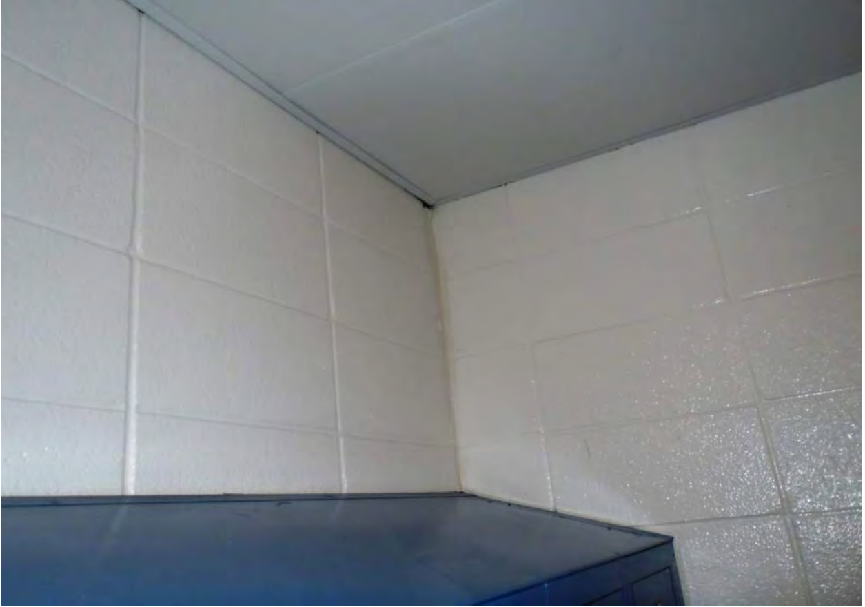
Photo 9A - Masonry Wall Cracking at Locker Room
