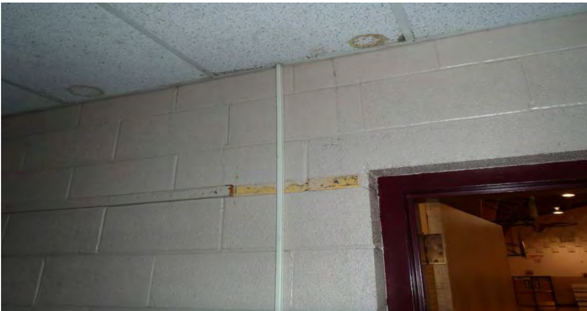
Photo 2B - Minor Settlement Crack at Interior Non-Bearing Masonry Wall
