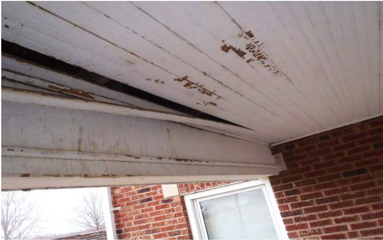
Photo 4E - West Deck Deterioration
