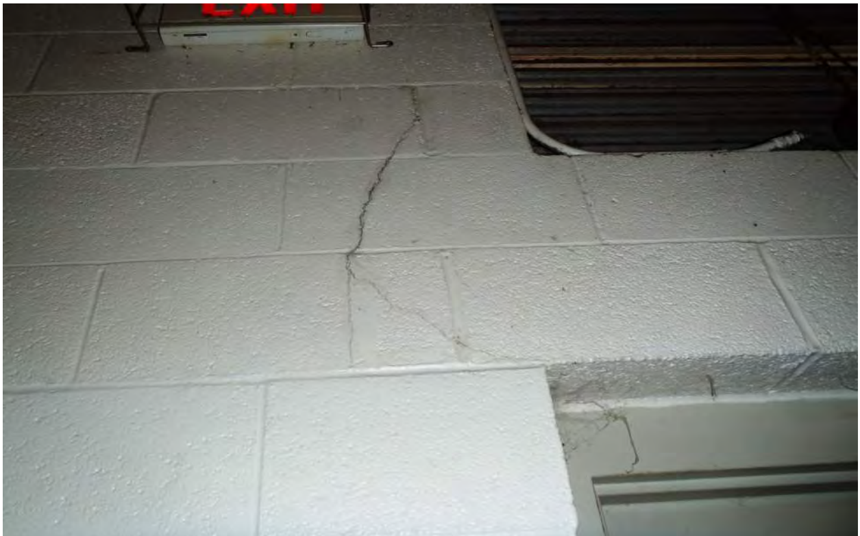
Photo 7C - Significant Wall Crack at Mechanical Room Masonry
