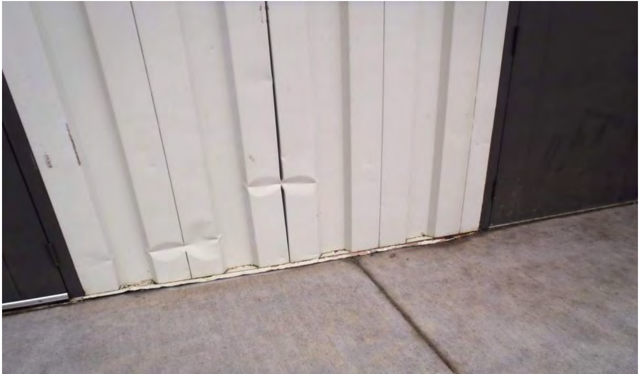
Photo 1A - Metal Facade Panel Impact Damage
