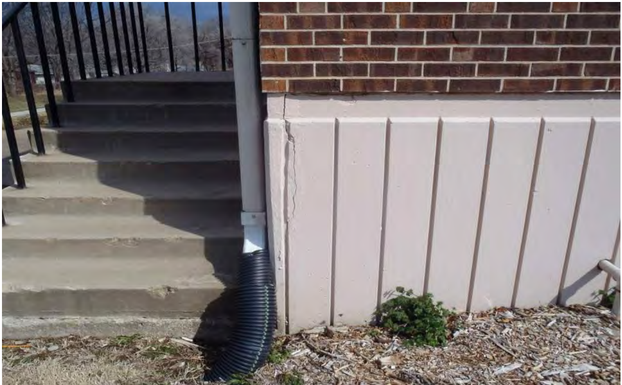
Photo 7F - Concrete Crack / Spall at Lower Level
