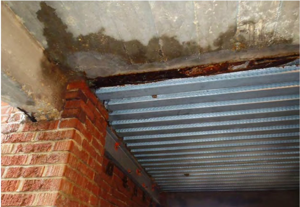
Photo 4K - Deterioration at South Exterior Concrete
