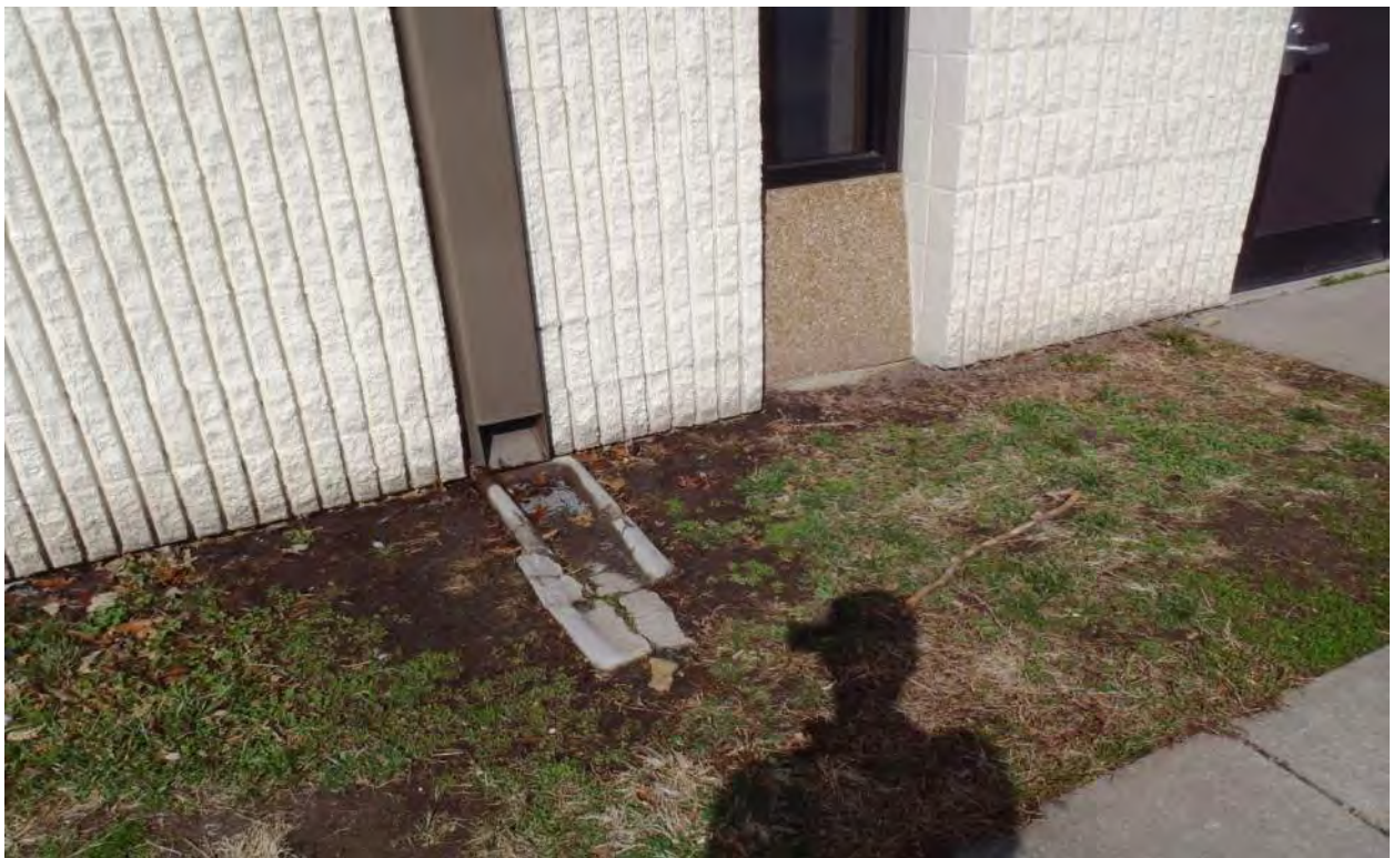
Photo 6C - Downspout Adjacent to Building
