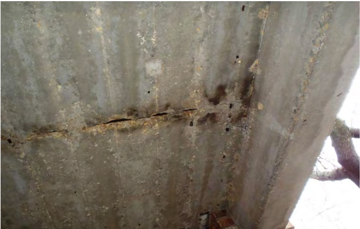
Photo 4O - Corrosion Deterioration at South Exterior Concrete
