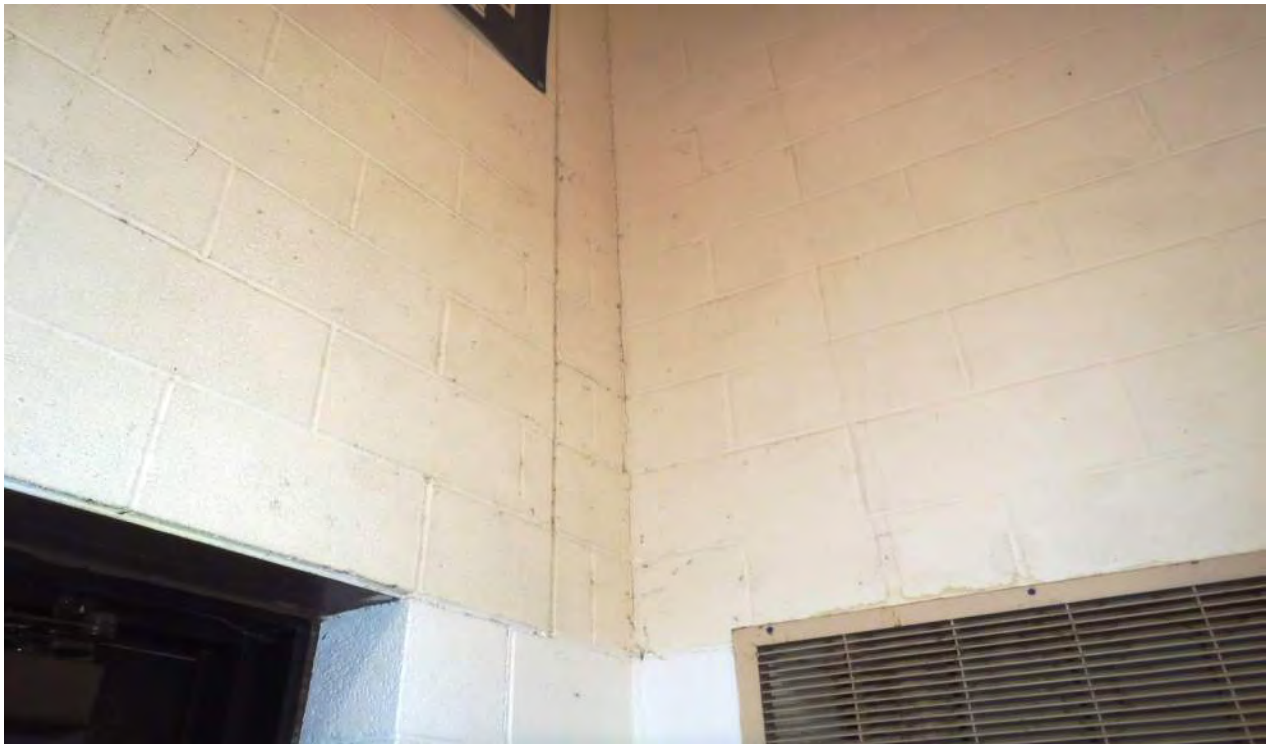
Photo 3C - Masonry Cracking at Interior Gymnasium Wall
