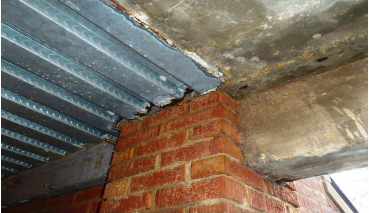
Photo 4L - Deterioration at South Exterior Concrete
