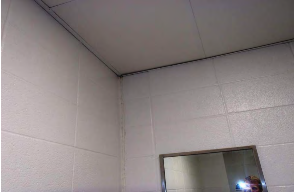
Photo 9B - Masonry Wall Cracking at Locker Room
