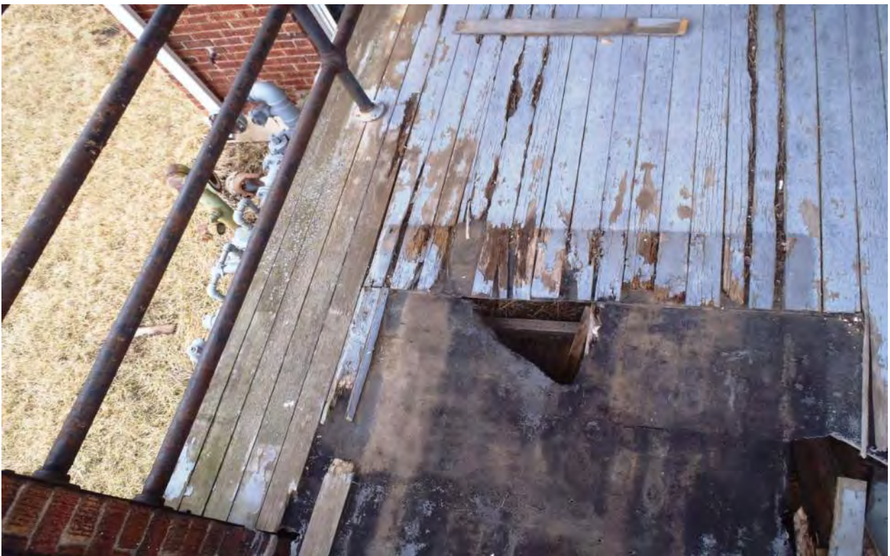
Photo 4H - West Deck Deterioration
