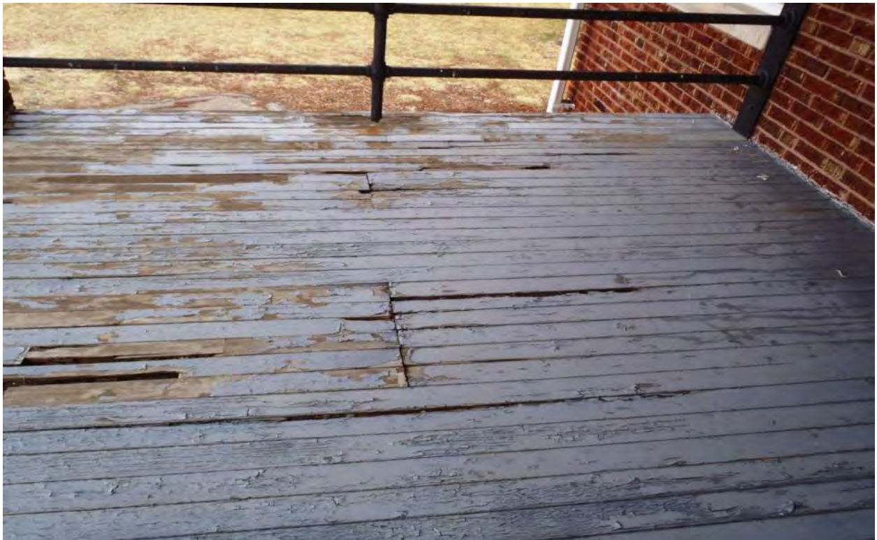
Photo 4B - West Deck Deterioration
