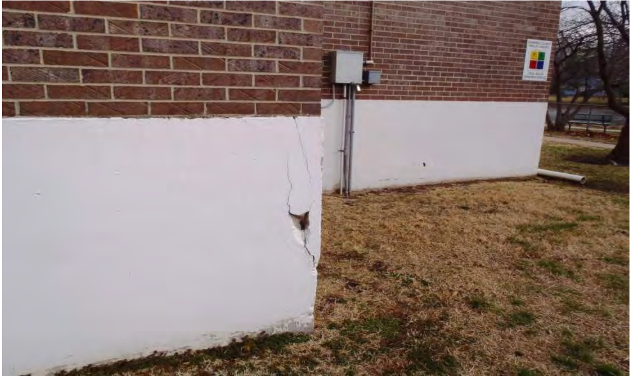
Photo 3D - Concrete Spalling at Exterior Concrete Structure
