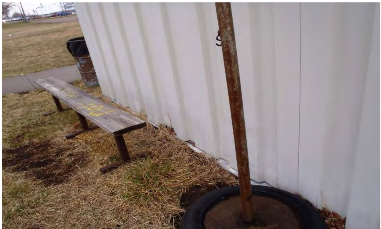
Photo 1C - Metal Facade Panel Impact Damage
