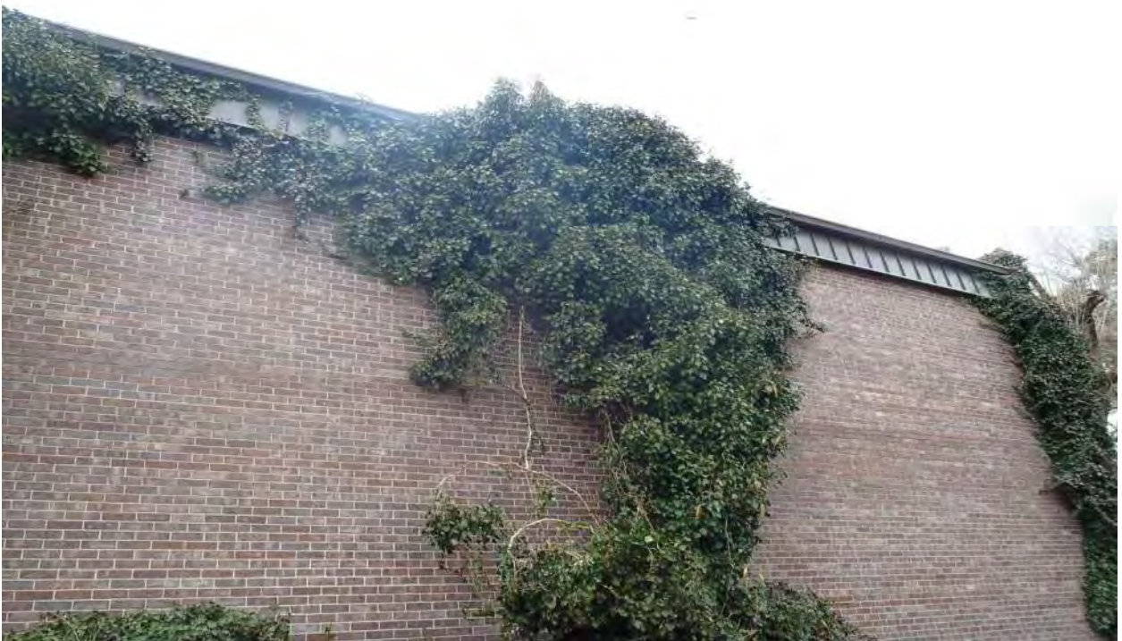
Photo 8C - Vegetation Growing on Structure
