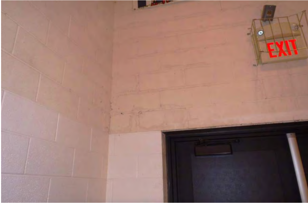
Photo 3B - Masonry Cracking at Interior Gymnasium Wall
