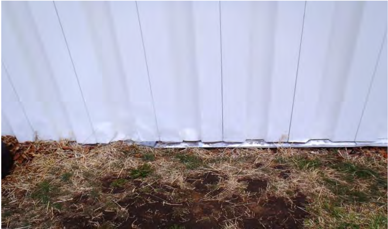
Photo 1D - Metal Facade Panel Impact Damage
