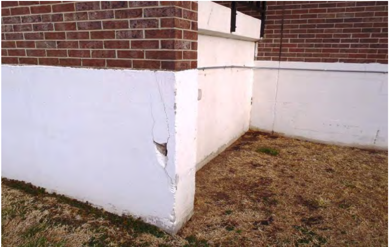
Photo 3E - Concrete Spalling at Exterior Concrete Structure
