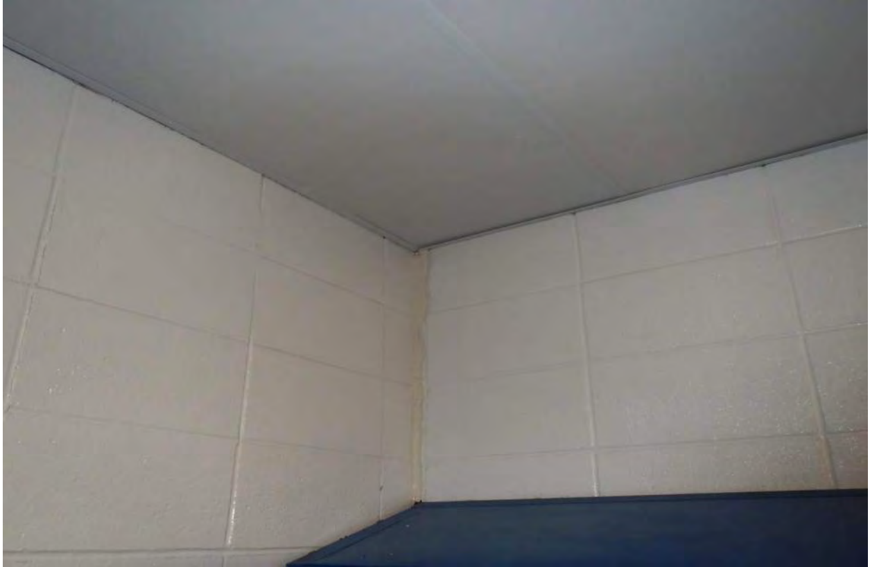
Photo 9D - Masonry Wall Cracking at Locker Room
