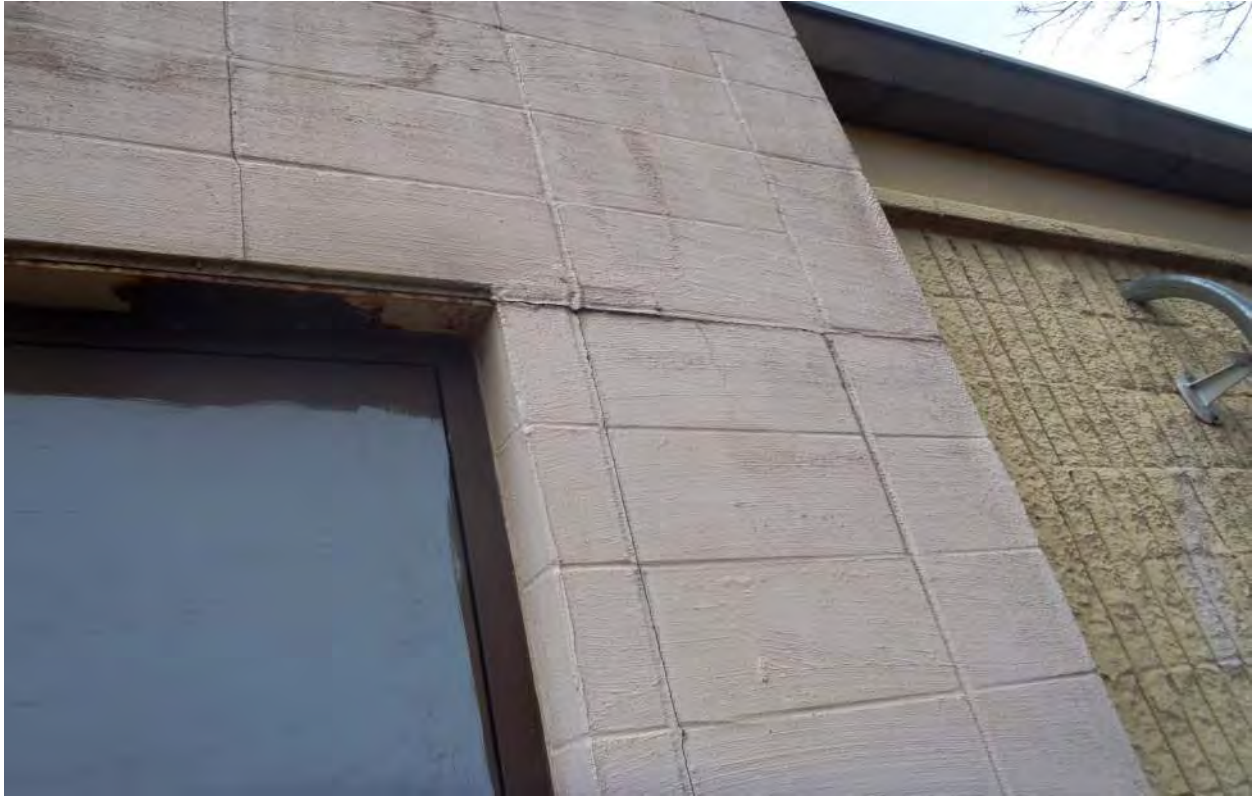
Photo 9G - Exterior Masonry Cracking
