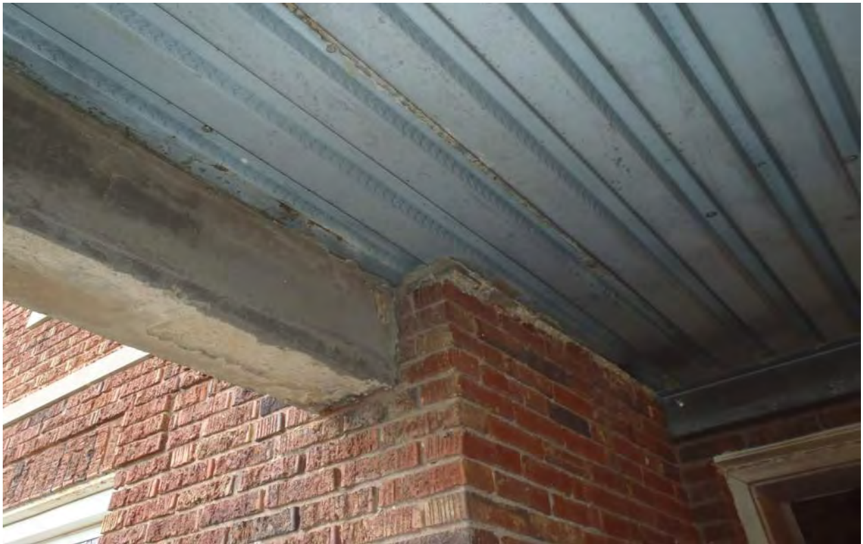
Photo 4M - Corrosion Deterioration at South Exterior Concrete
