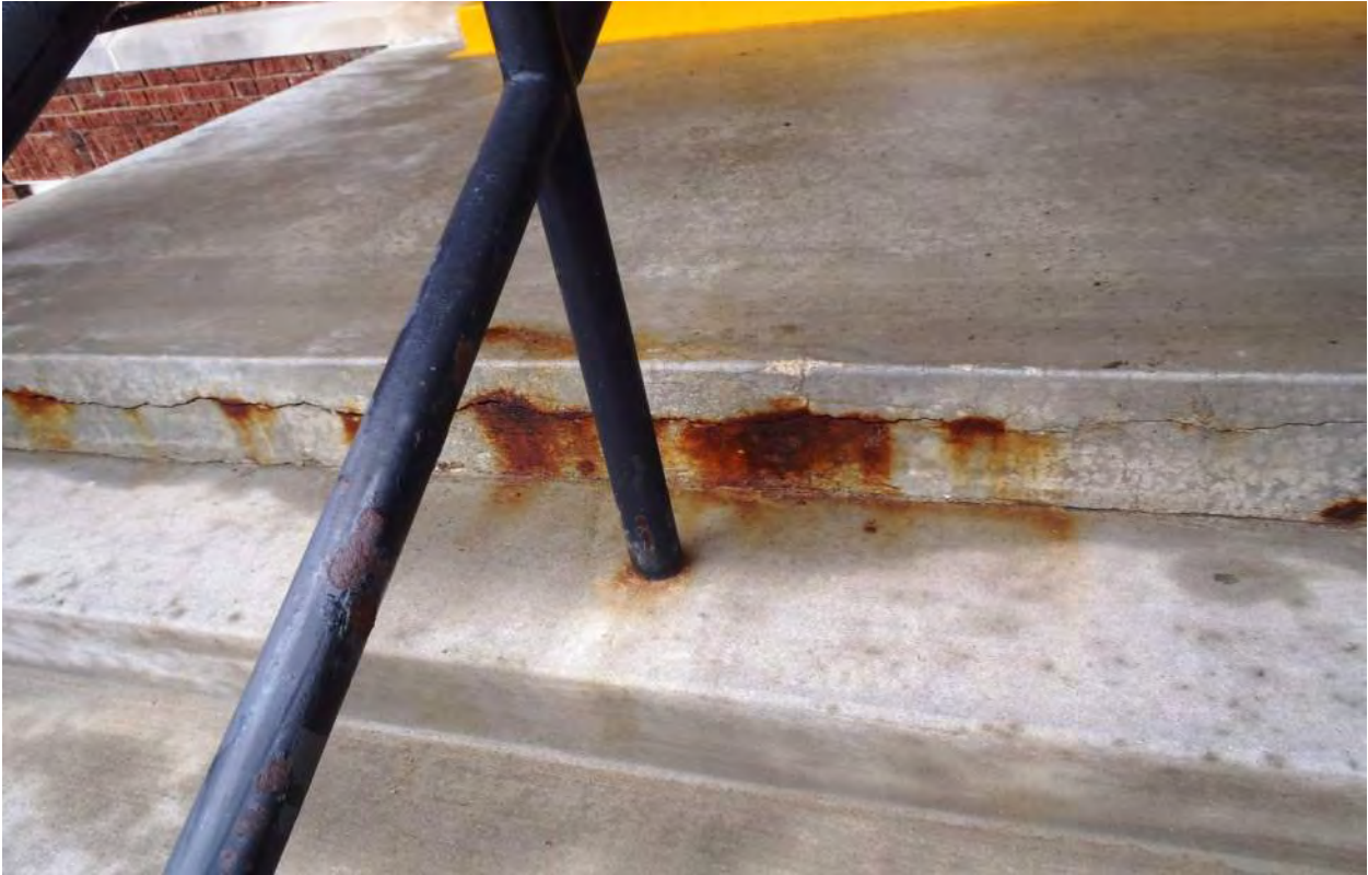
Photo 4N - Corrosion Deterioration at South Exterior Concrete
