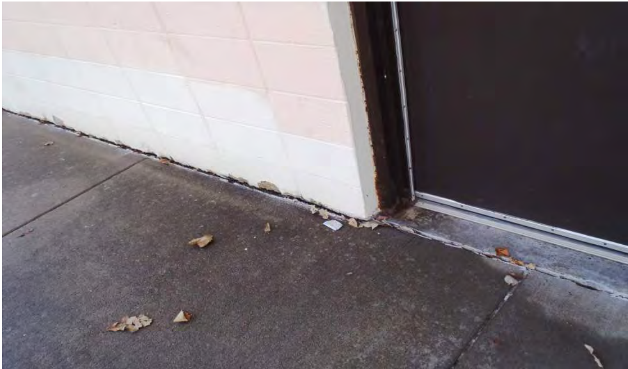
Photo 6D - Exterior Concrete Spalling
