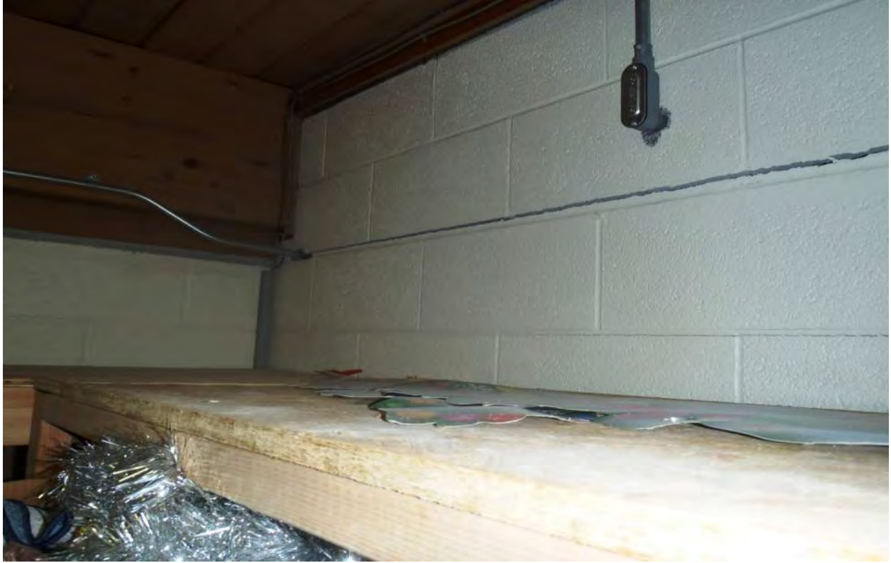
Photo 7B - Significant Wall Crack at Mechanical Room Masonry
