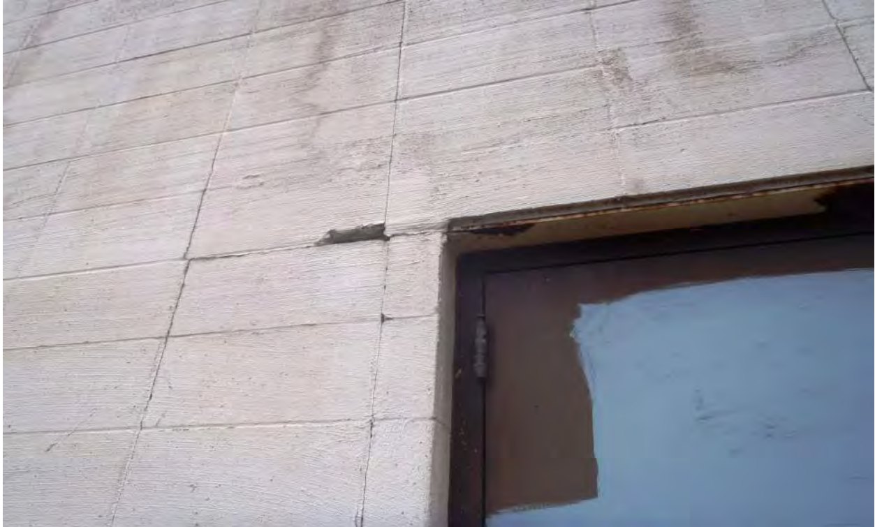
Photo 9F - Exterior Masonry Cracking
