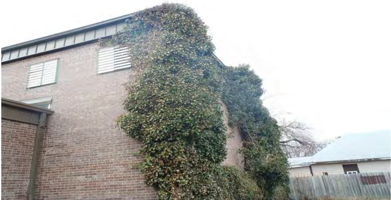
Photo 8A - Vegetation Growing on Structure
