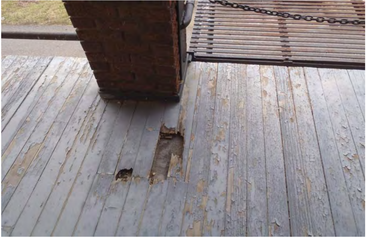
Photo 4A - West Deck Deterioration
