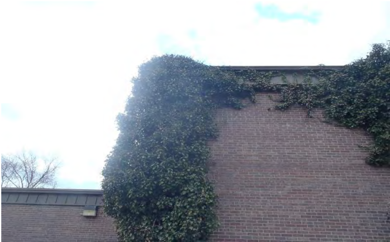
Photo 8D - Vegetation Growing on Structure
