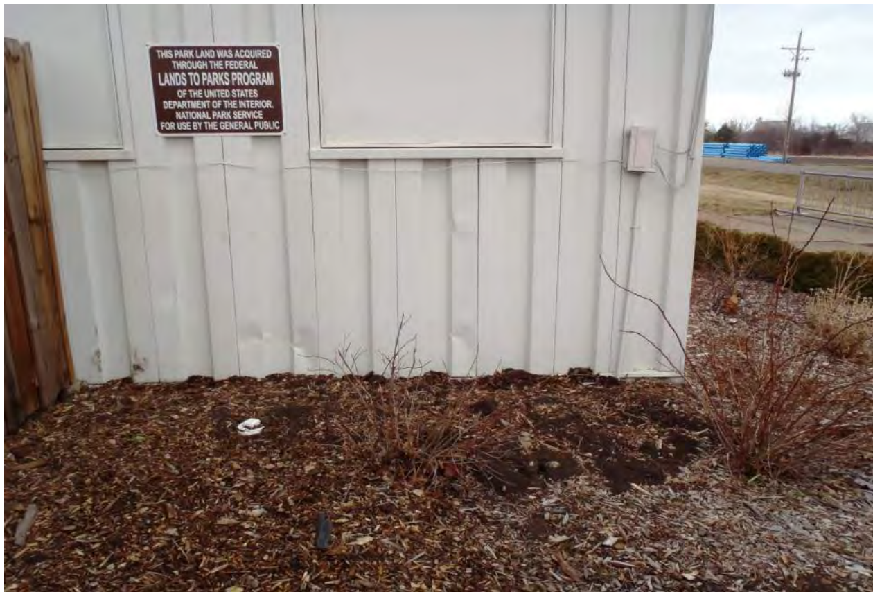
Photo 1B - Metal Facade Panel Impact Damage
