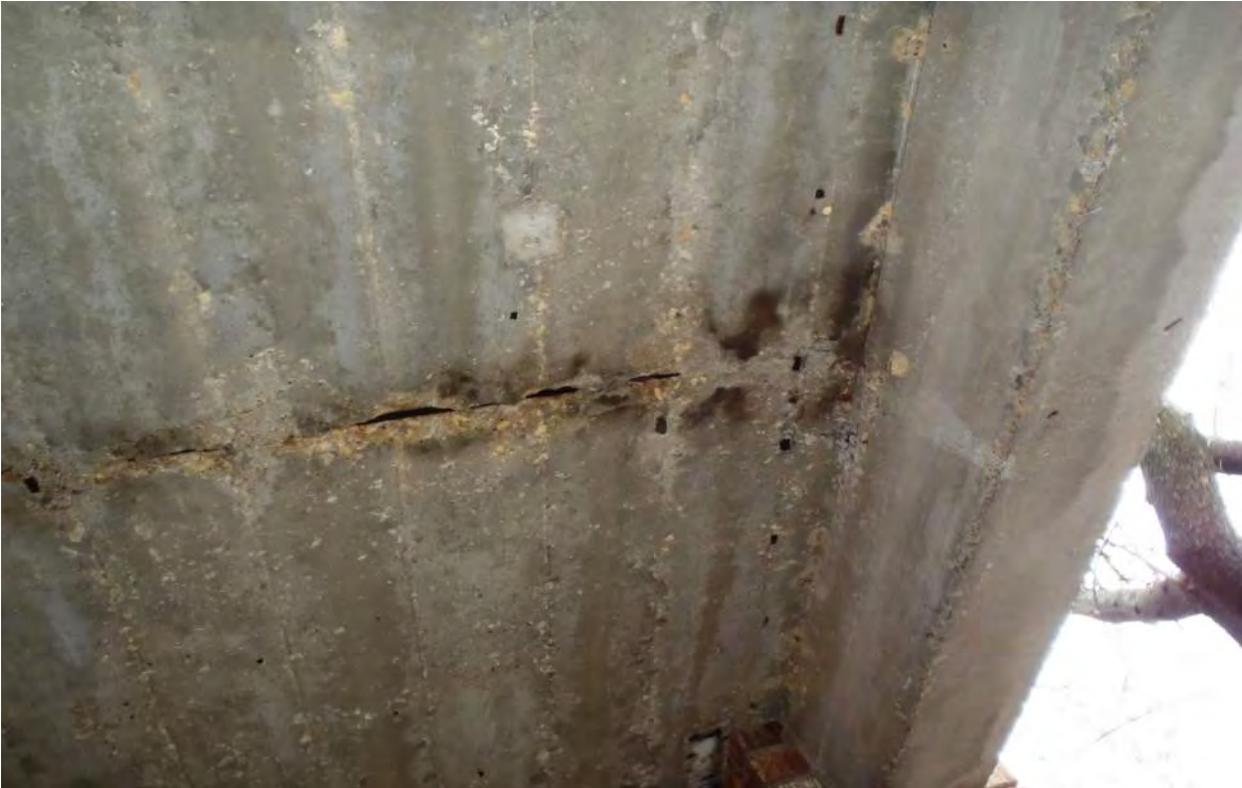
Photo 4O - Corrosion Deterioration at South Exterior Concrete
