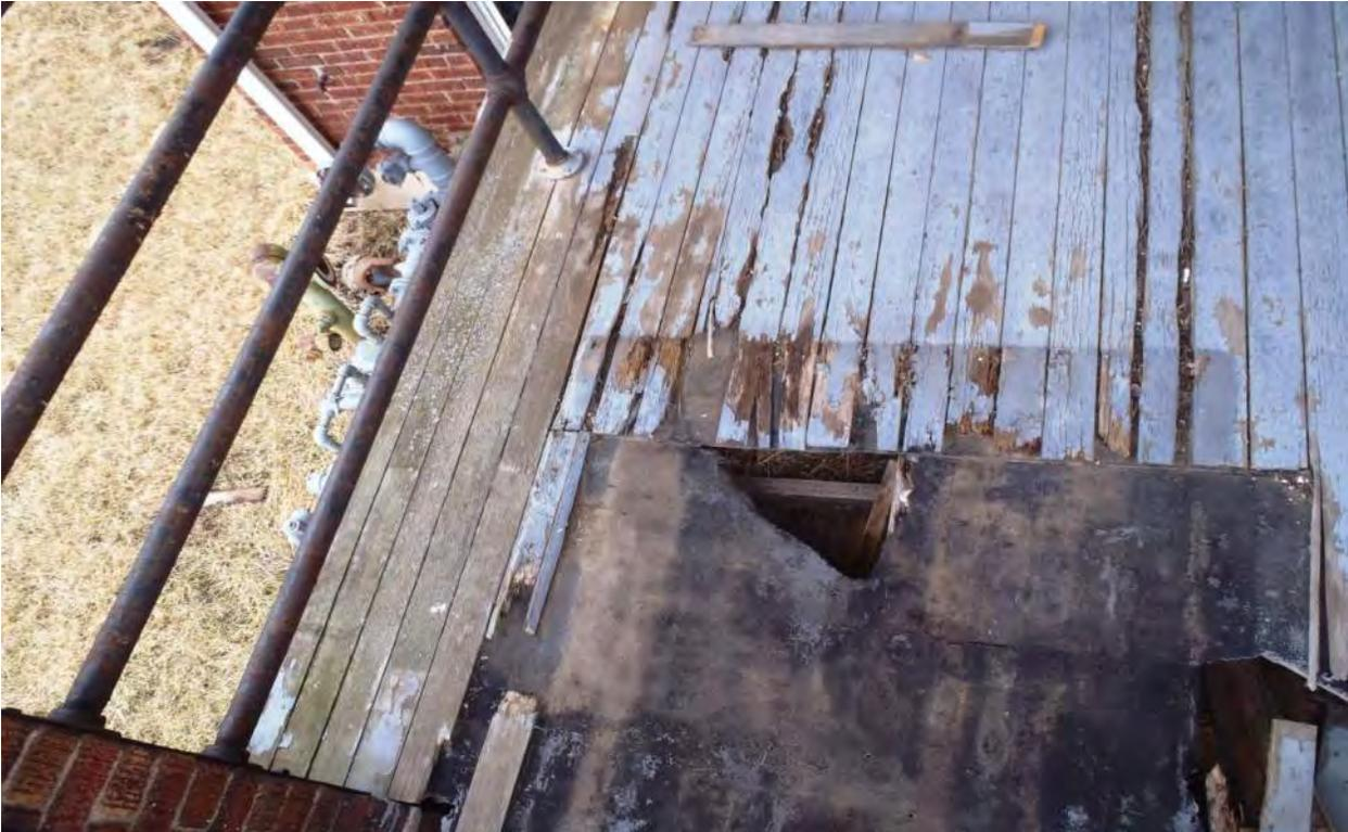
Photo 4H - West Deck Deterioration
