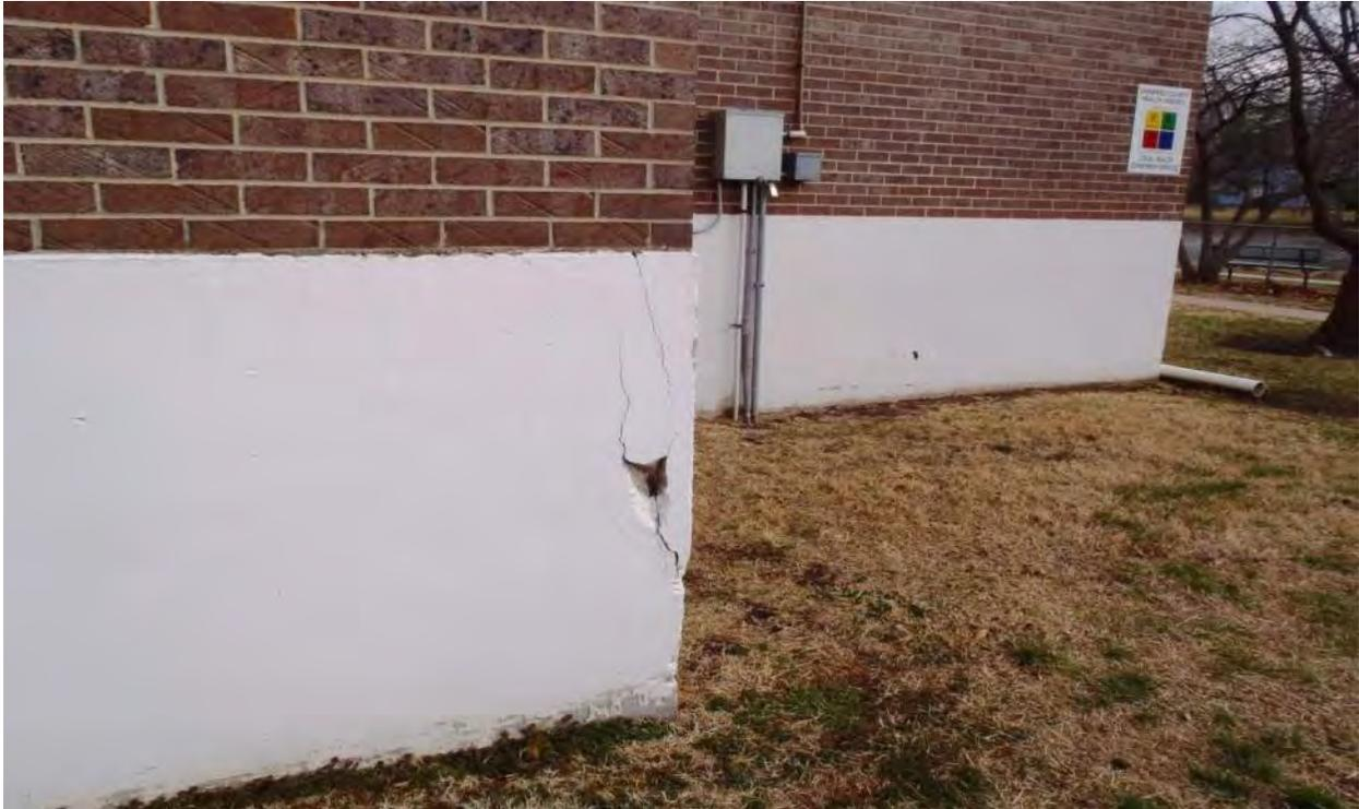
Photo 3D - Concrete Spalling at Exterior Concrete Structure
