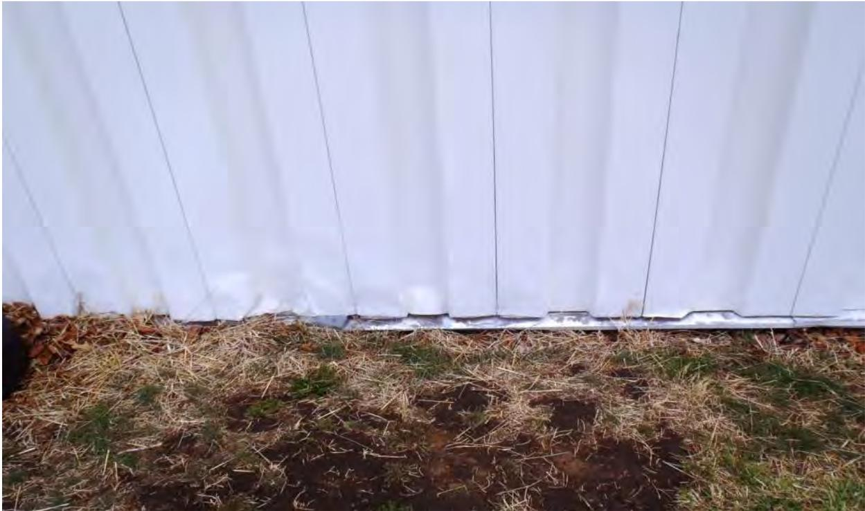
Photo 1D - Metal Facade Panel Impact Damage
