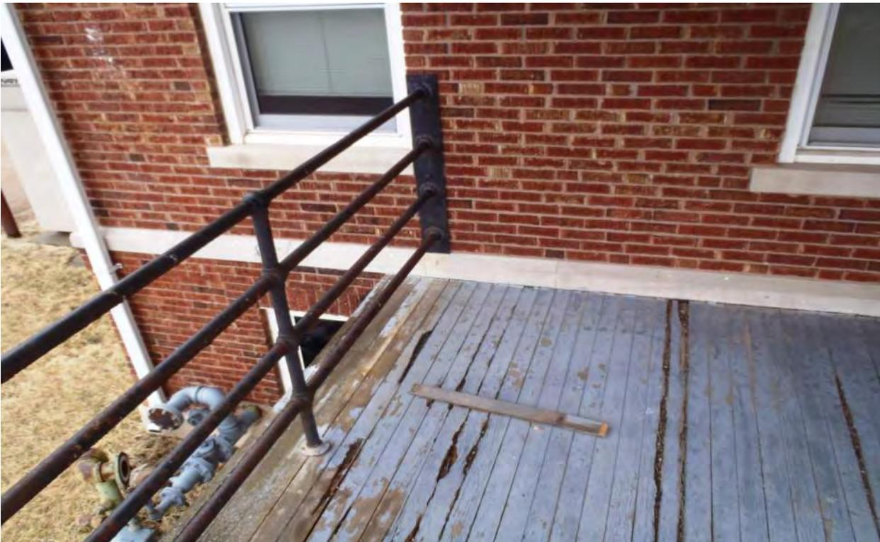
Photo FG - West Deck Deterioration
