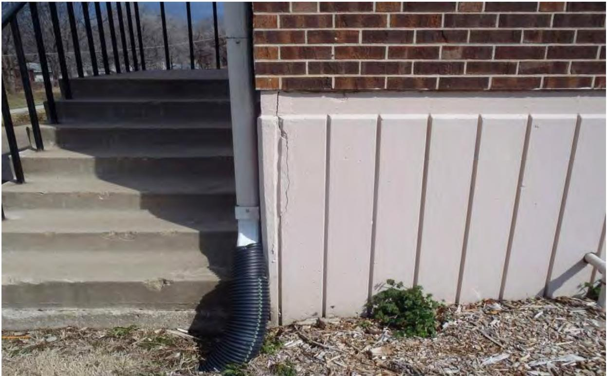
Photo 7F - Concrete Crack / Spall at Lower Level
