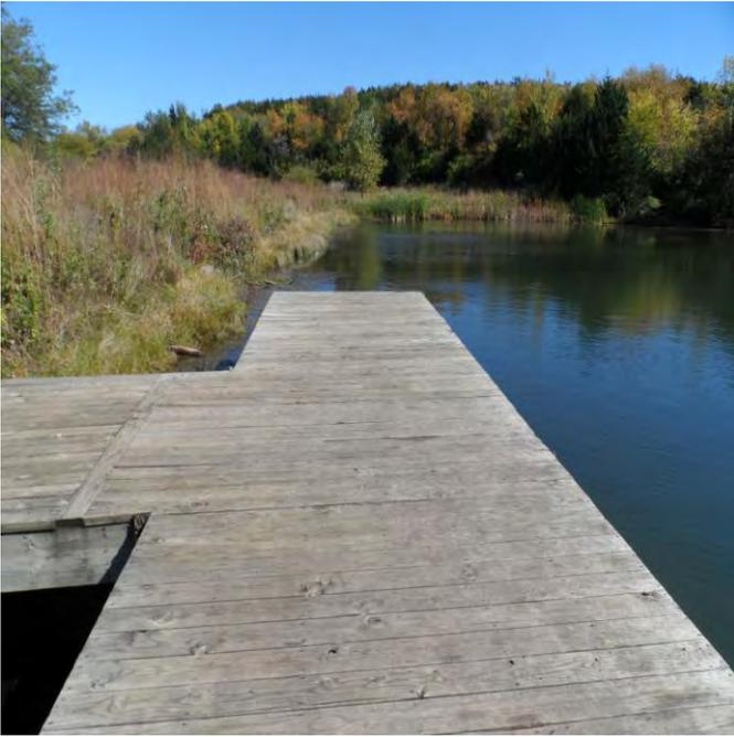
**Image 5:** Decking of the fishing dock is in general good condition, however railing around the dock is missing.
