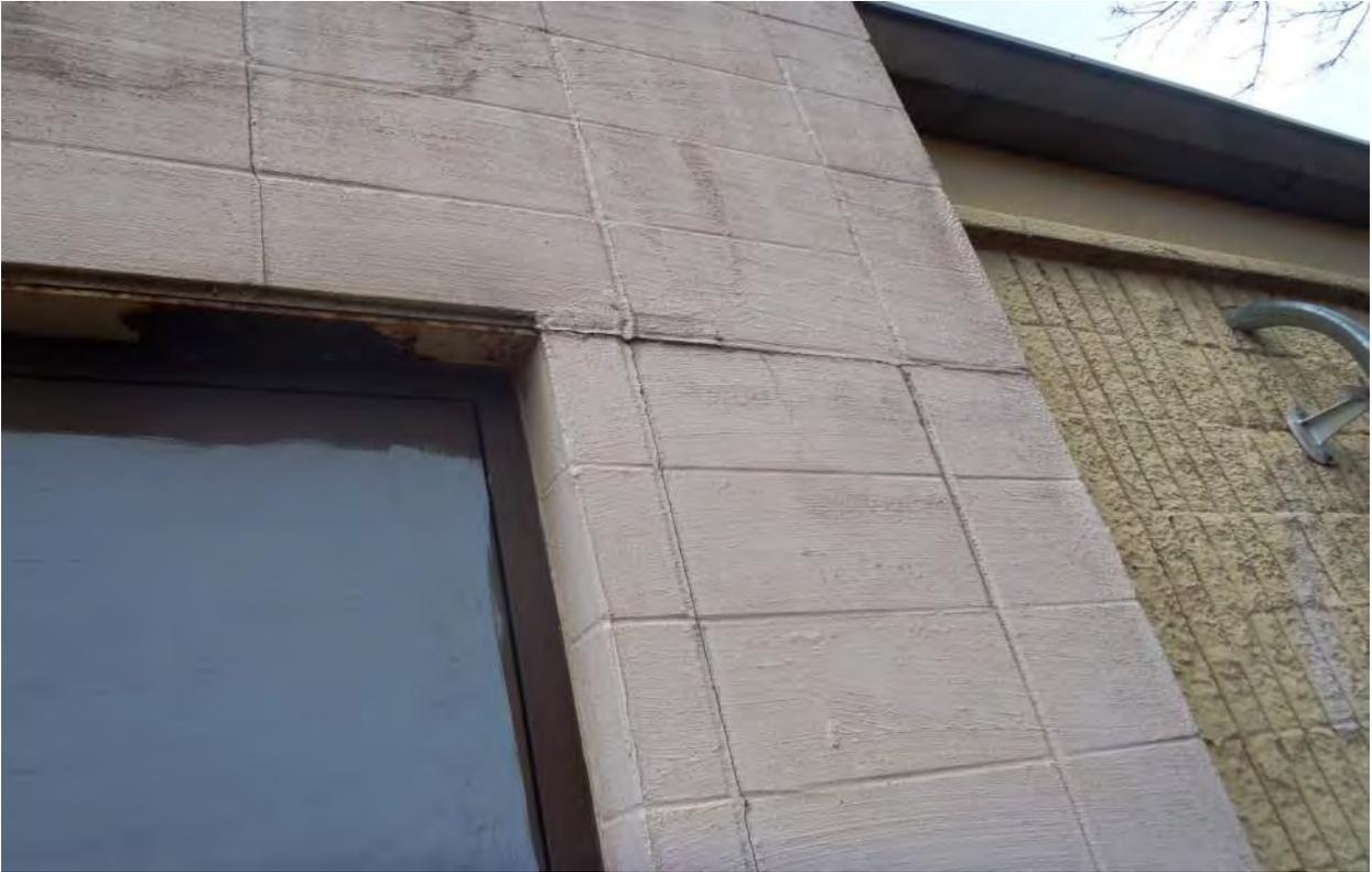
Photo 9G - Exterior Masonry Cracking
