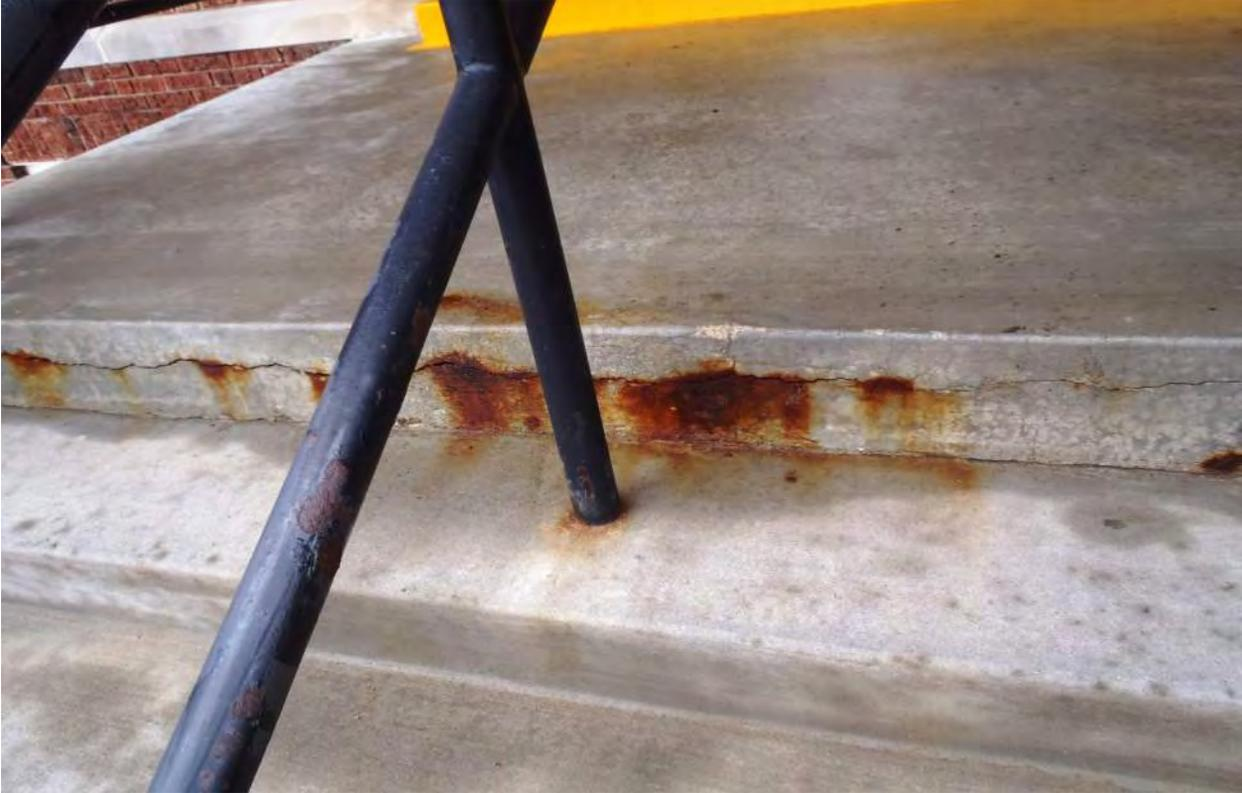
Photo 4N - Corrosion Deterioration at South Exterior Concrete
