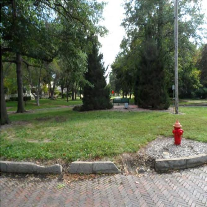
**Image 5:** Some of the islands show deterioration of the stone curb. Others have recently had their stone curbs repaired.
