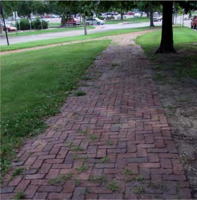
**Image 1:** Brick pavers are in good condition, but need to be reset
