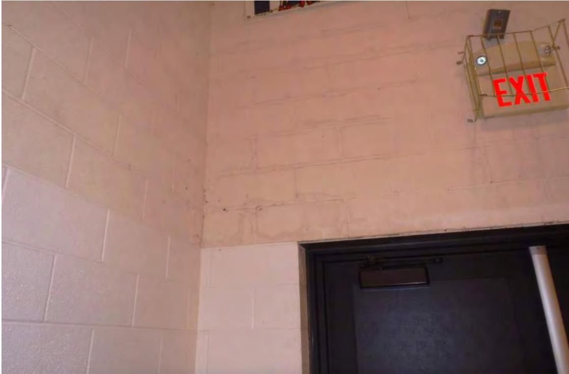
Photo 3B - Masonry Cracking at Interior Gymnasium Wall
