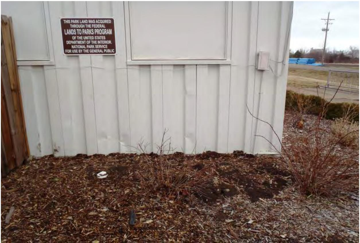
Photo 1B - Metal Facade Panel Impact Damage
