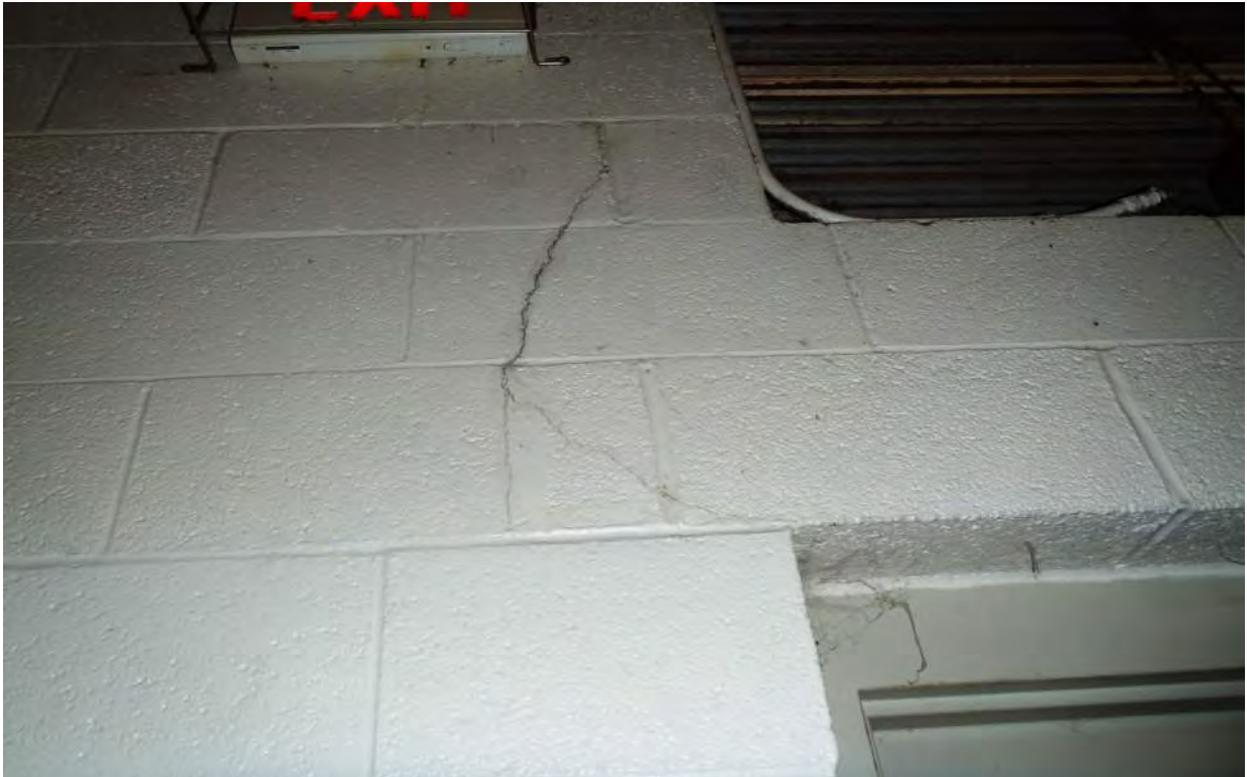
Photo 7C - Significant Wall Crack at Mechanical Room Masonry
