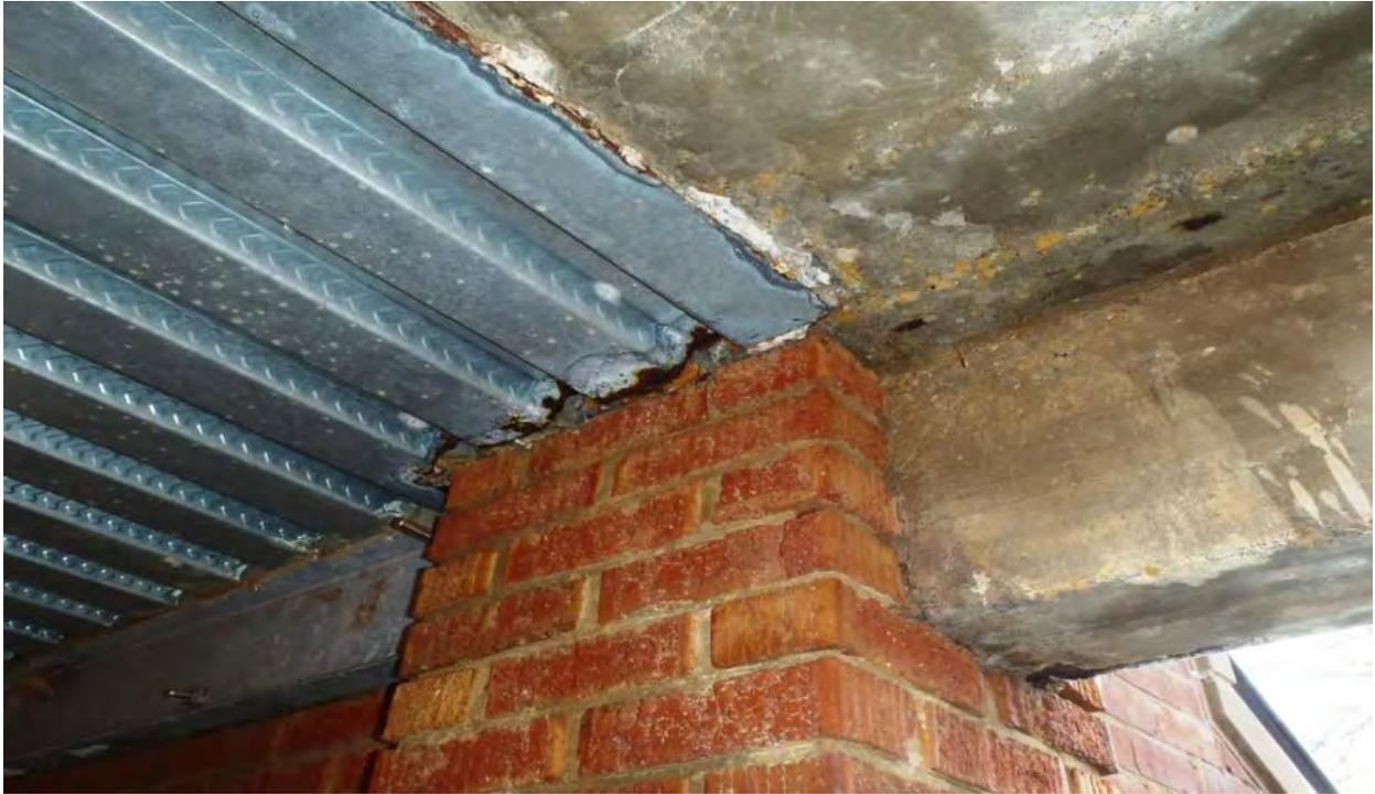
Photo 4L - Deterioration at South Exterior Concrete
