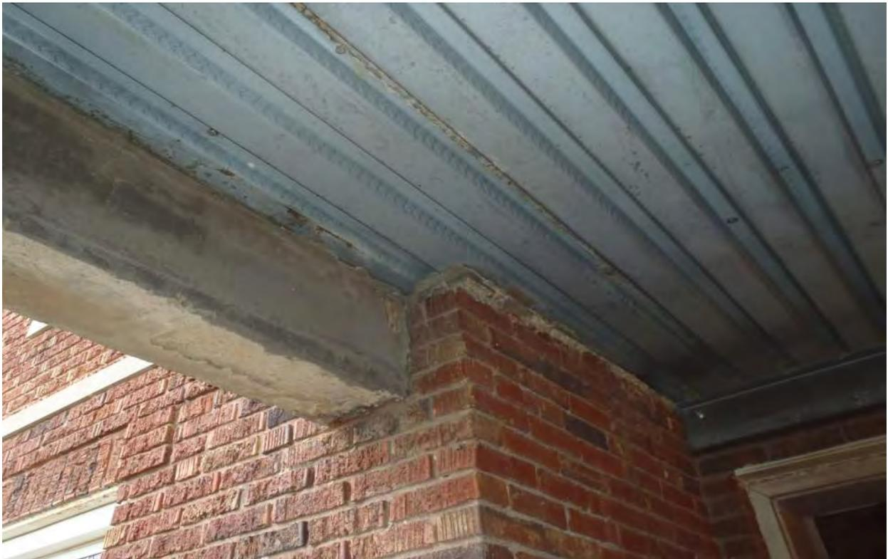
Photo 4M - Corrosion Deterioration at South Exterior Concrete
