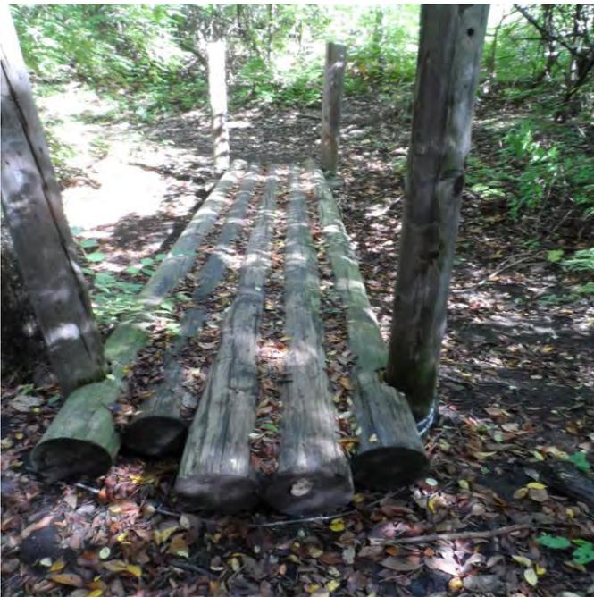
**Image 7:** Rough handmade bridge that spans a low water crossing.
