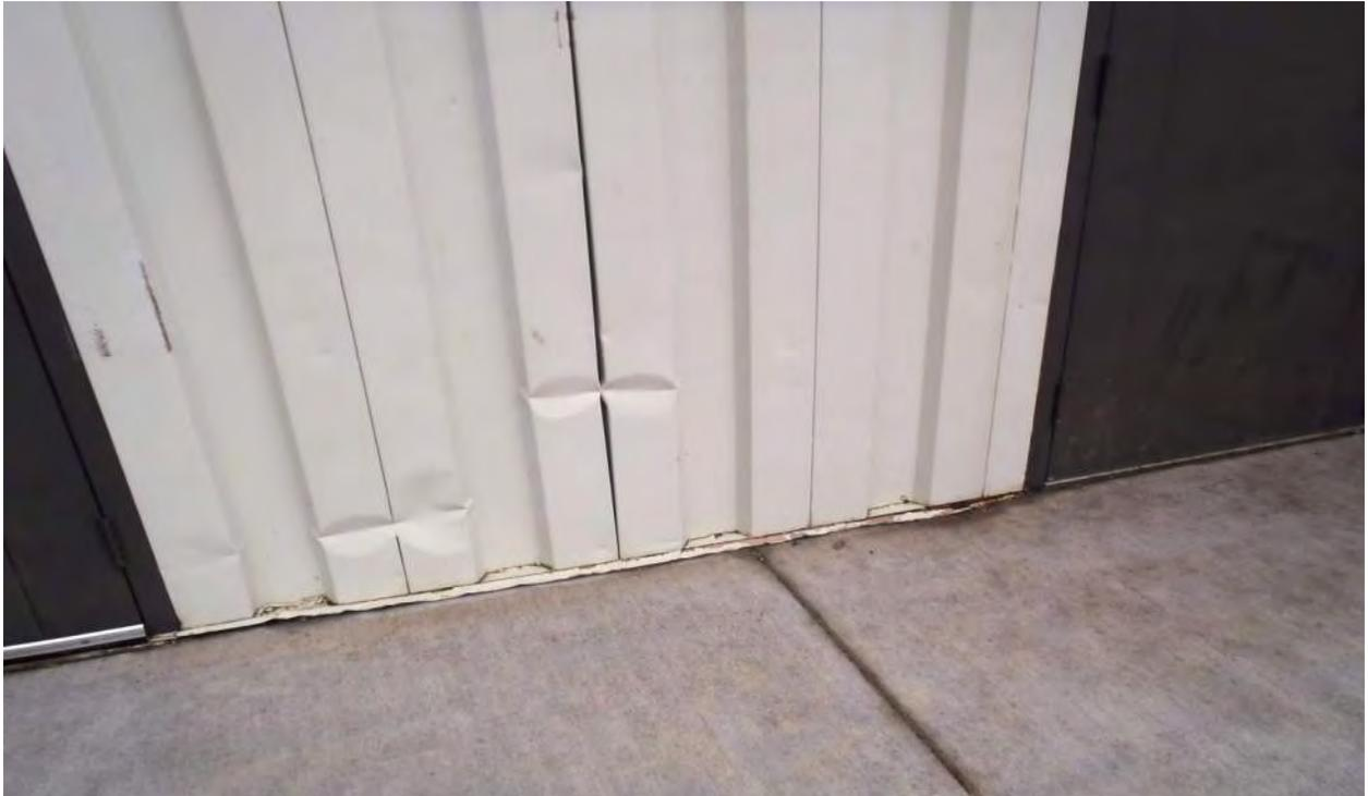
Photo 1A - Metal Facade Panel Impact Damage
