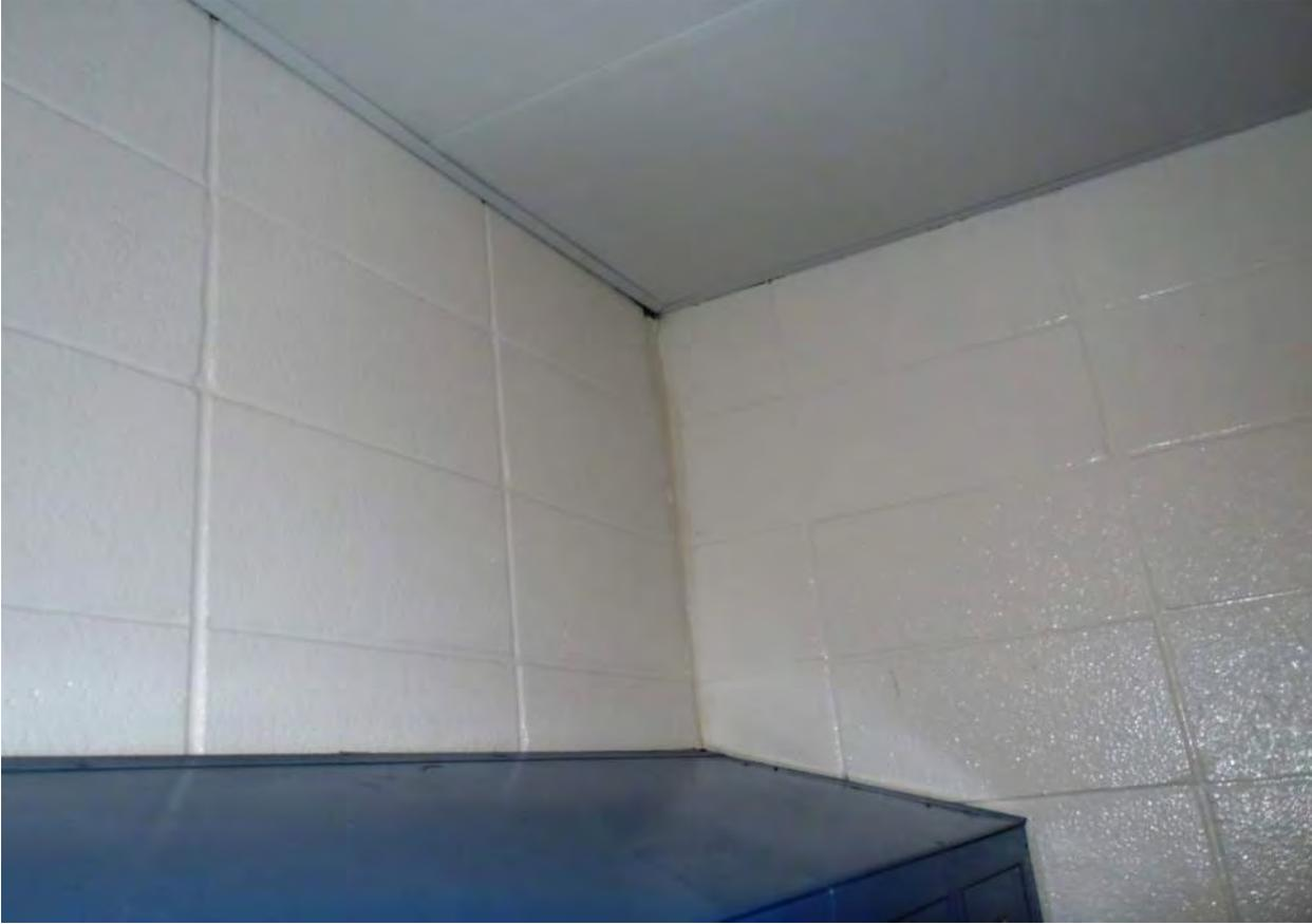
Photo 9A - Masonry Wall Cracking at Locker Room
