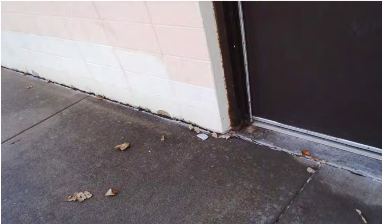
Photo 6D - Exterior Concrete Spalling
