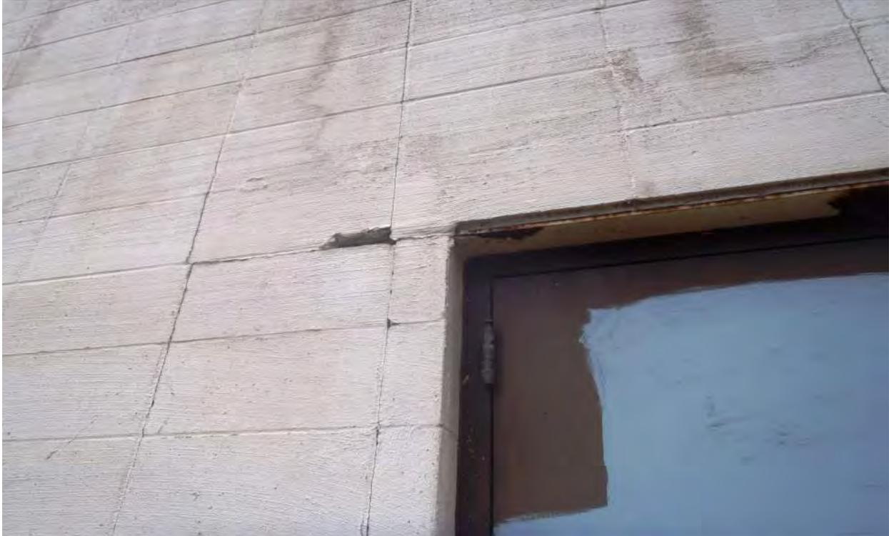
Photo 9F - Exterior Masonry Cracking
