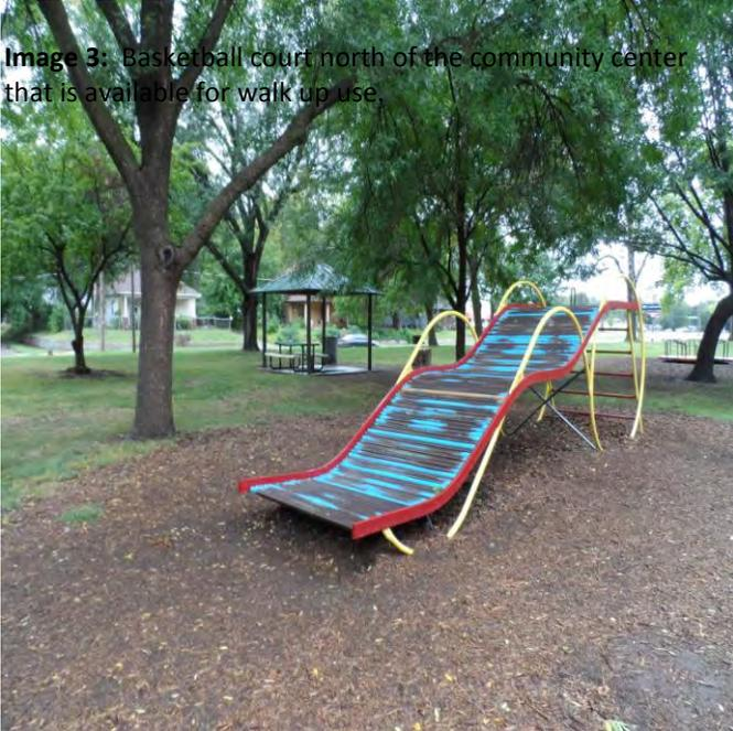
**Image 5:** Roller slide that is fun but does not meet current standards. No fall surface or accessible route.
