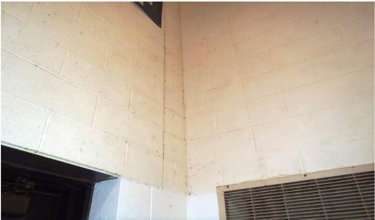
Photo 3C - Masonry Cracking at Interior Gymnasium Wall
