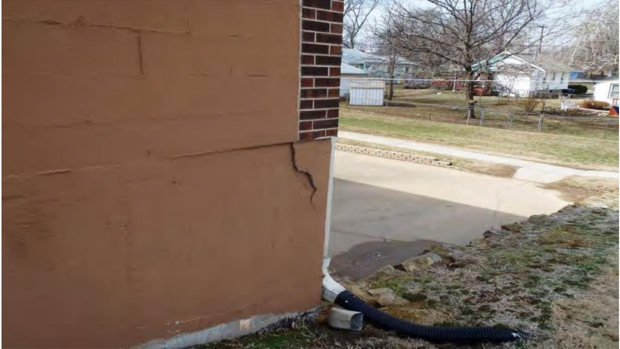
Photo 7E - Concrete Crack / Spall at Lower Level
