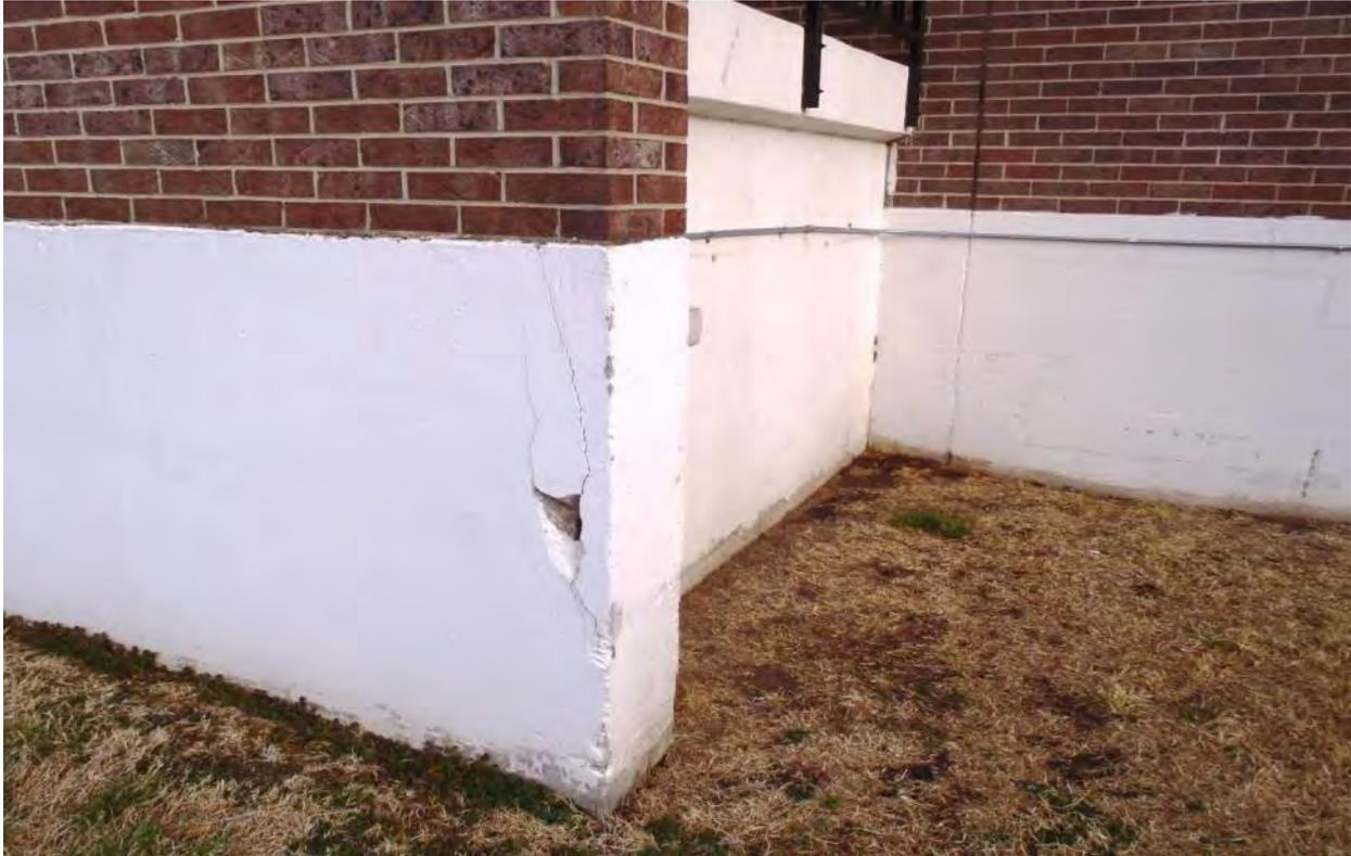
Photo 3E - Concrete Spalling at Exterior Concrete Structure
